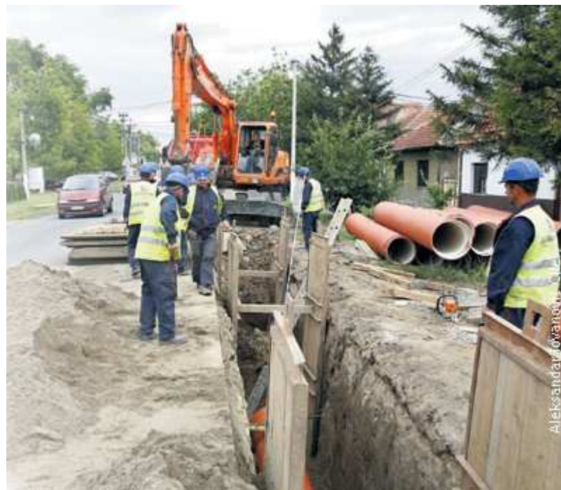
Excavation for pipelines
