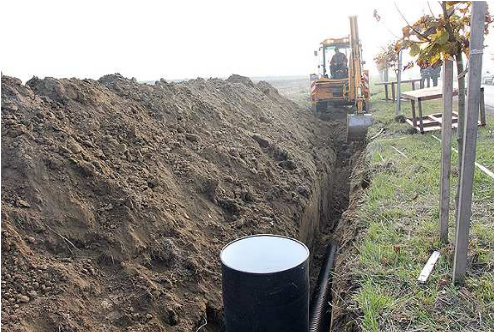
Industrial Sewerage network in Lajkovac, PVC pipes
