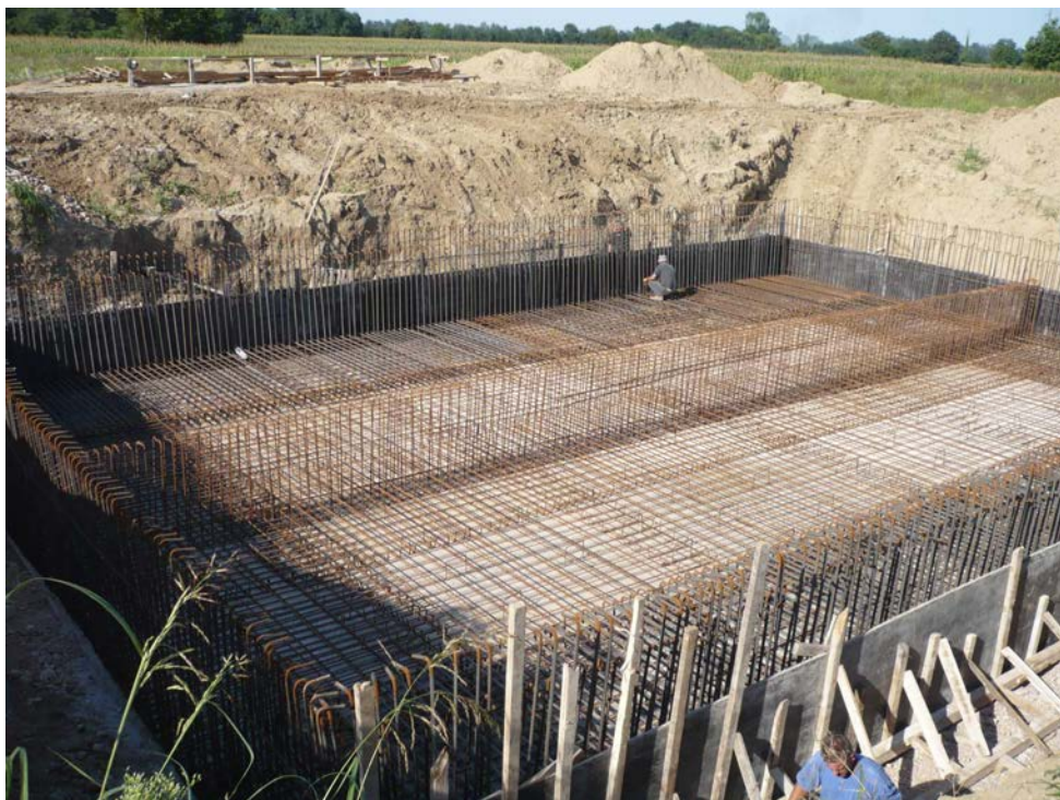
Waste water treatment plant Reinforcement for bottom slab of aeration tank
