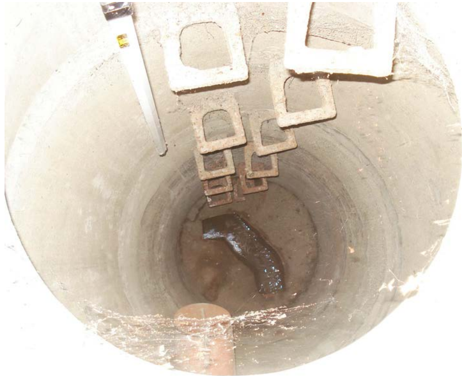
Sewerage network manhole
