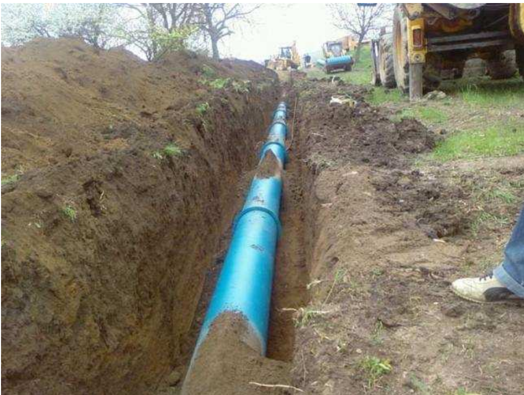
Industrial Sewerage network in Lajkovac, PVC pipes
