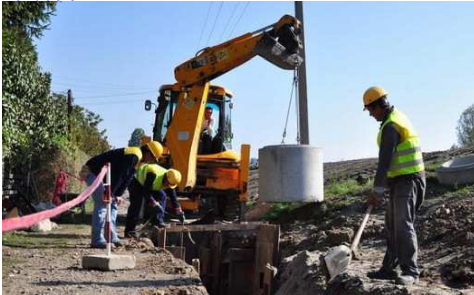
Industrial Sewerage network in Lajkovac, montage manholes
