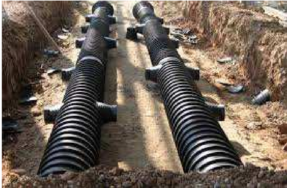
PE corrugates Sewerage network pipeline
