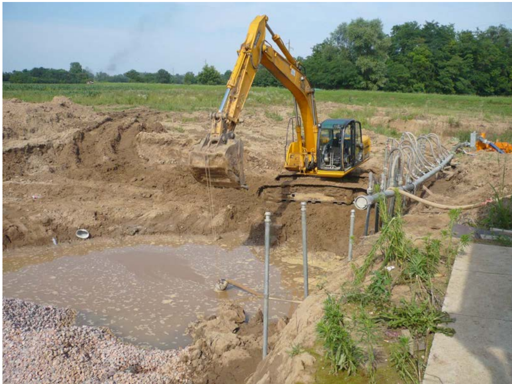
Wide excavation for waste water treatment plant with needle filters
