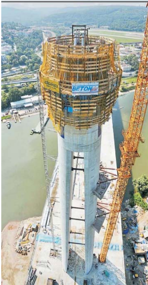
March 2010 Poured 13th pylon segment - west leg and installing reinforcement for 14th segment - east leg
