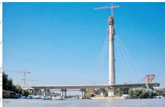
Sept 2010 - Back and Main span with 12 stayed cables connected to pylon
