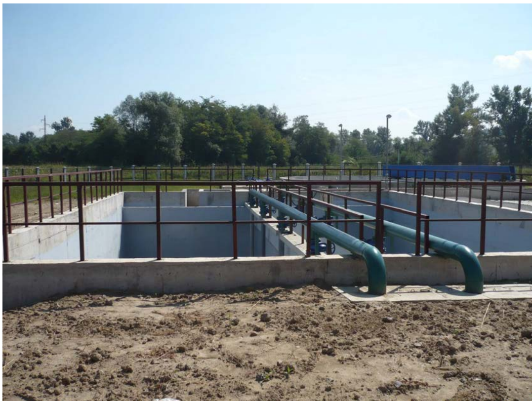
Waste water treatment plant Aeration tank in final phase
