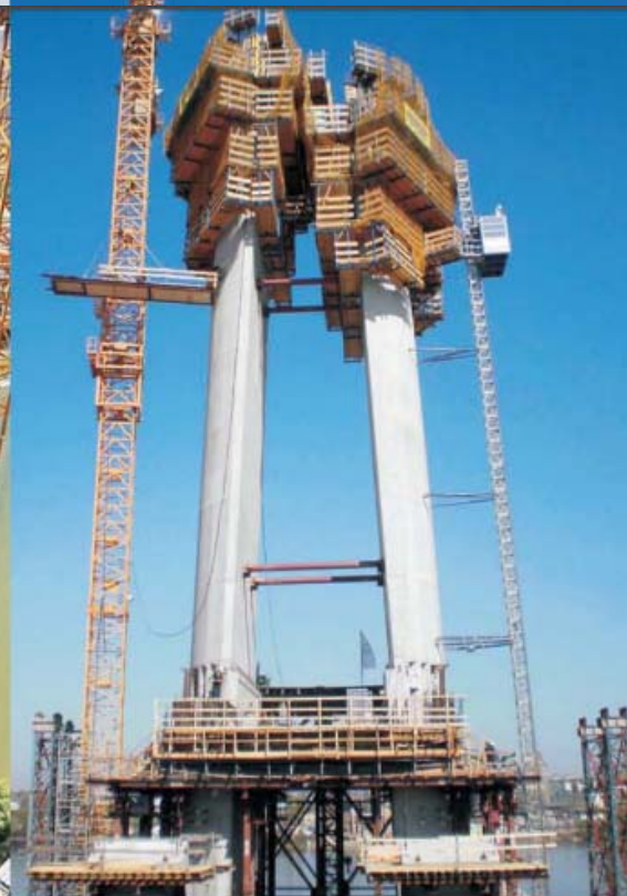
March 2010 Poured 13th pylon segment - west leg and installing reinforcement for 14th segment - east leg
