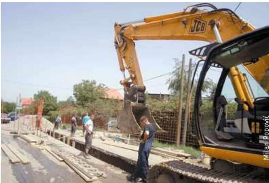
Industrial Sewerage network in Lajkovac, montage manholes
