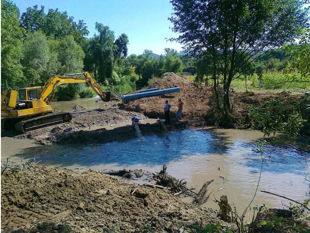
Crossing PVC sewerage with passing barrier ,Nikola Tesla Power plant
